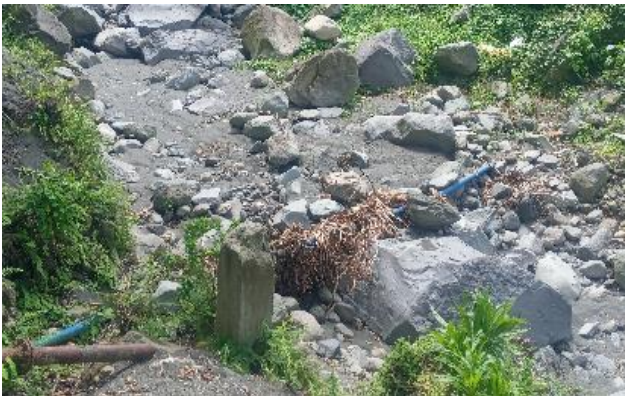
Owia. Note pipe is on river bed and vulnerable to damage from any loose boulders or other objects from further upstream. Easy to access by persons.
