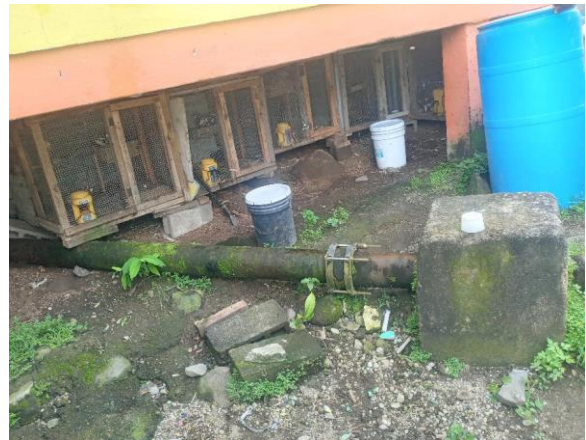
Closer view of pipe crossing under residence. Limited space to facilitate any maintenance or construction work. Issue of noise and dust. Domestic birds in cages under house.
