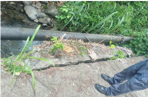
Crossing on way to Perseverance Water Treatment Facility in Jennings. Water overtops bridge especially when culverts are blocked and has damaged bridge and threatens pipeline.
