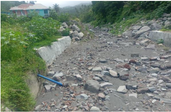
Another example of river crossing with pipe going under existing river bed.
