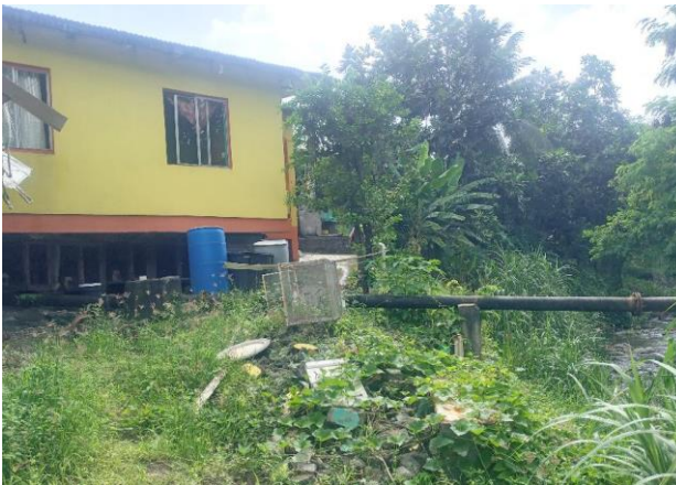
Concrete residence has been constructed over the 6" dia water pipeline on the banks of the Perseverance River at Spring Village where it crosses the river..
