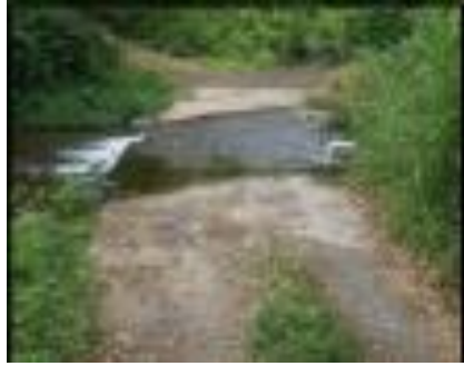
Figure 4. Photo of a river crossing along the Jennings Mountain Road +930
