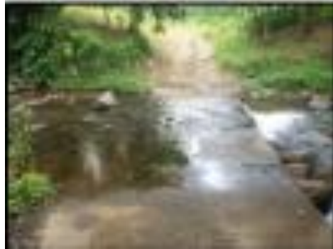
Figure 5. Photo of a river crossing along the Jennings Mountain Road 1+060
