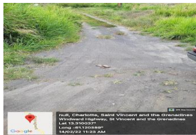
Figure 3. Photo showing road section of Waterloo # 3 road (0+412).
