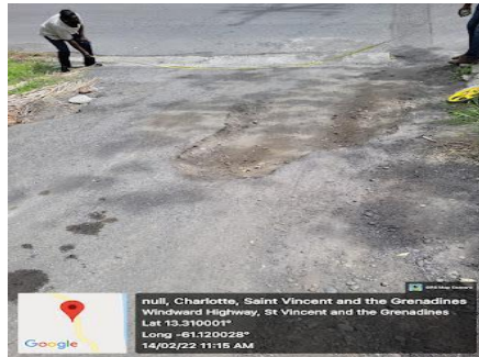
Figure 2. Photo showing the start of waterloo #3 road (0+000)
