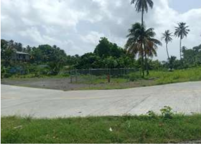
Borehole BHD site at Overland Magnum. View of existing fenced area enclosing the capped existing test borehole. Site is flat. Note proximity of residents to the north across the riverbed. Existing Highway provided easy access to the site.
