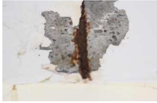
Heavily corroded embedded reinforcement.
