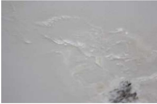
Signs of water penetration in roof slab.
