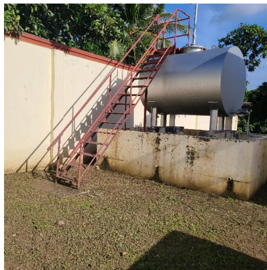
Above ground diesel storage tank with secondary containment. The tank is not covered and the drainage outlets from the containment are not plugged.
