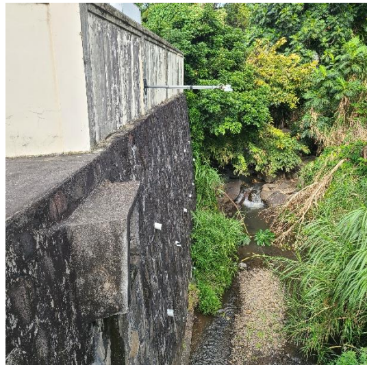
River wall on NEMO's south boundary. Note drainage outfall in foreground and river gauge apparatus mounted on the wall. The opposite riverbank is vegetated.
